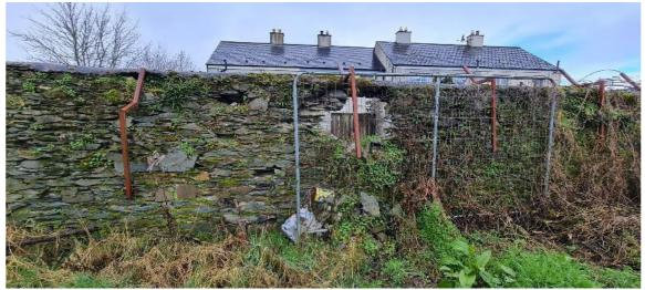
Fig. 15 Collapsed area of masonry on the south boundary wall of Tanyard
