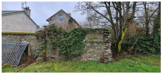
Fig. 8 Detail of the west boundary wall incorporating the west wall of an earlier (now demolished) building.
