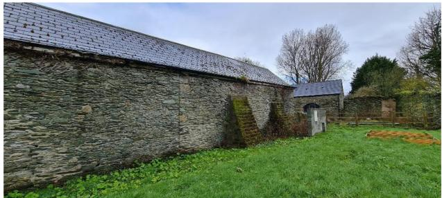
Fig. 6 Rear (east) façade of Building No. 2, showing vertical joint between two phases of construction and stone rubble buttresses at north end of building. The enclosed yard to the east of the building includes raised planting beds, recently used for the planting of vegetables.
